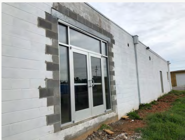
The new door to the Refuge Community Center.
